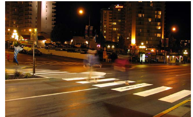
Example of continental pedestrian crosswalks. All pedestrian crosswalks in the City, including Manchester Road, should be continental style crosswalks.
