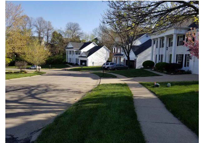
Existing residential sidewalk in Ballwin.
