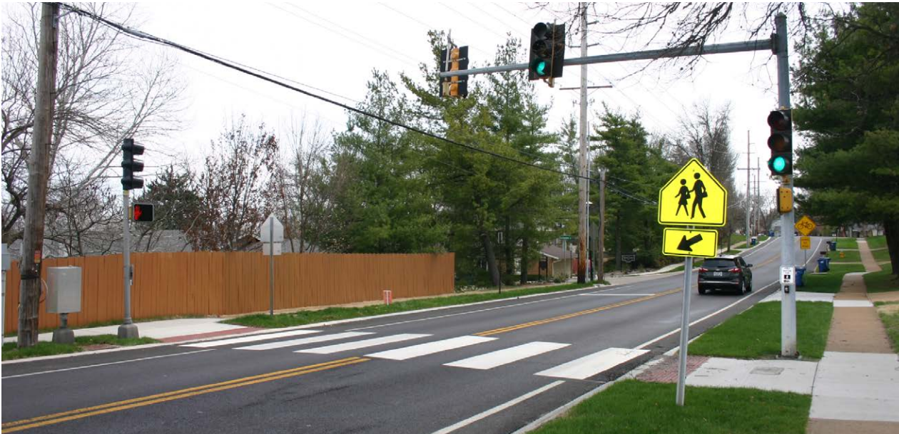
Existing mid-block crossing along Henry Avenue near Henry Elementary School. This mid-block crossing is already enhanced with a pedestrian-actuated signal. Other existing mid-block crossings in Ballwin should be evaluated for enhancements with a pedestrian-actuated signal or beacon (see Goal 2.6E).
