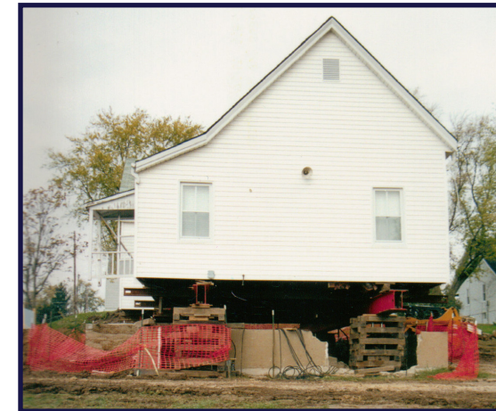
Photo: Old Ballwin Schoolhouse Move
