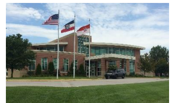
City of St. Charles, Police Station
