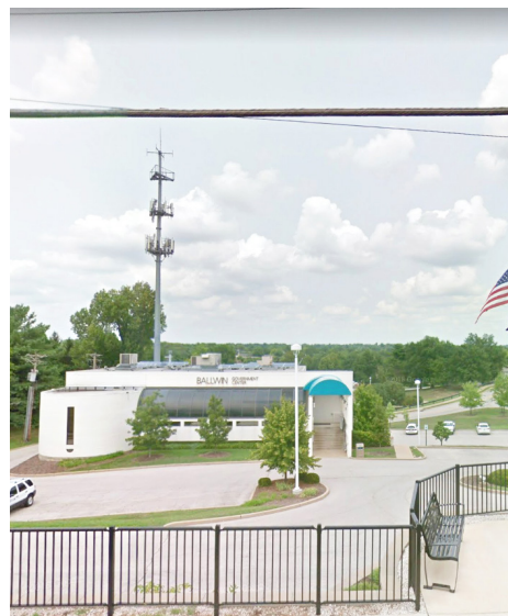
Existing City Hall
