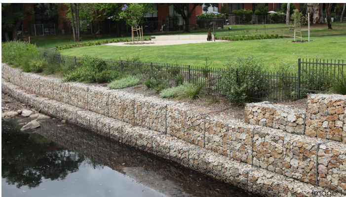
Gabion creek stabilization
