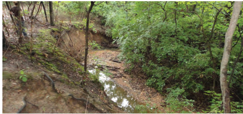
Existing Conditions at Ferris Park
