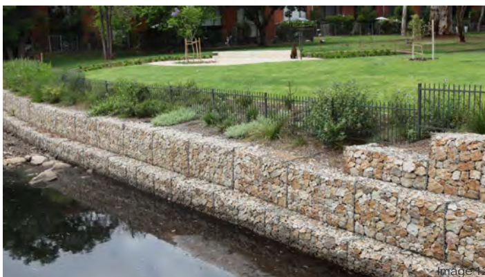
Gabion creek stabilization
