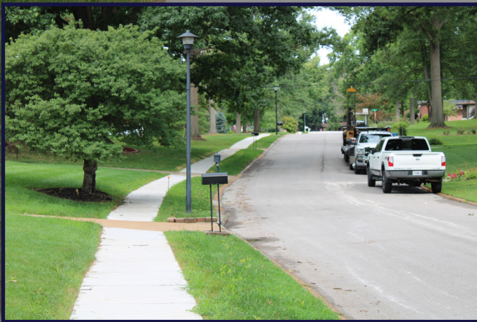
This sidewalk on Algonquin Drive from Kenilworth Lane to Claymont Drive was completed in June.
