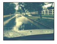
Kehrs Mill Road Ponding Remediation: Water ponds on Kehrs Mill Road in front of Essen Place subdivision. The ponding occurs after each rainfall and whenever the subdivision irrigation system is operating. To avoid utility conflicts, a slotted drain pipe would be installed under the curb and gutter and piped to a downstream curb
