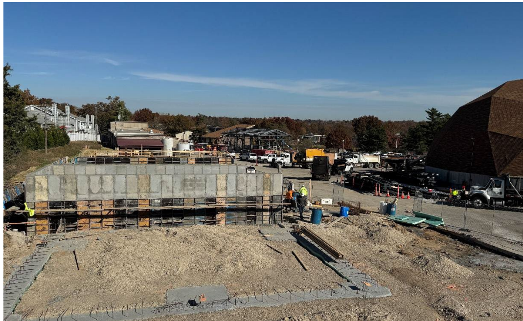
Public Works Yard under construction
