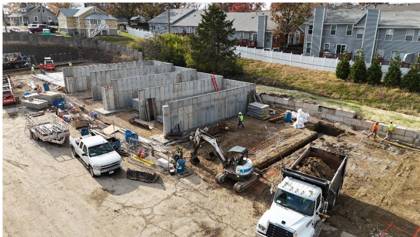
Public Works Yard new building site
