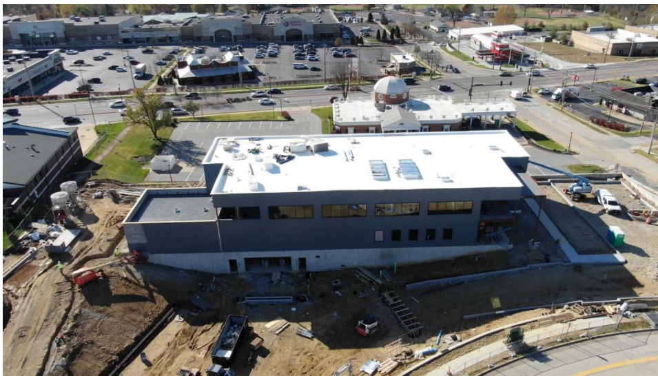
New Ballwin Police Station under construction
