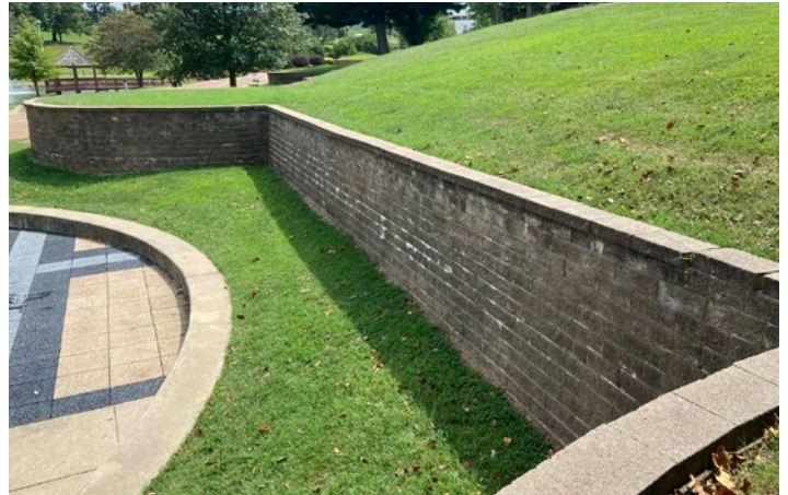
Figure 16: The large existing retaining wall currently creates an unwanted division within the park.
