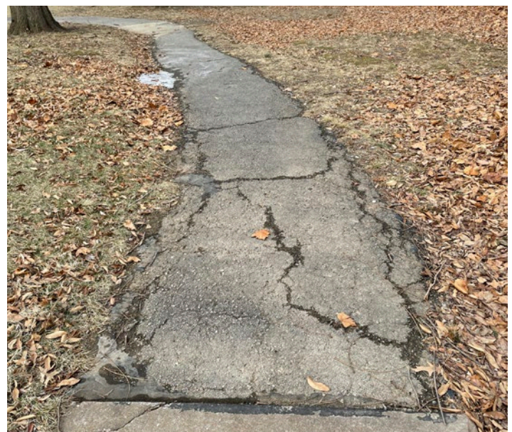
Figure 31: The asphalt path along the north side of the park creates a larger loop in the park but needs resurfacing.
