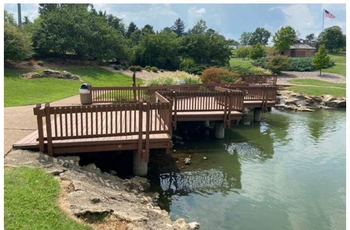
Figure 21: The decks on the south end of the lower pond are used by visitors for fishing and other activities but are deteriorating and require improvement or replacement.
