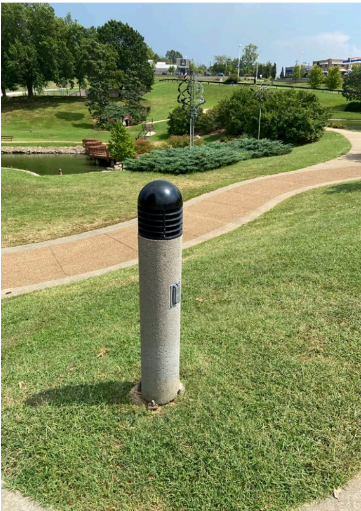
Figure 69: Light bollard with exposed aggregate finish.
