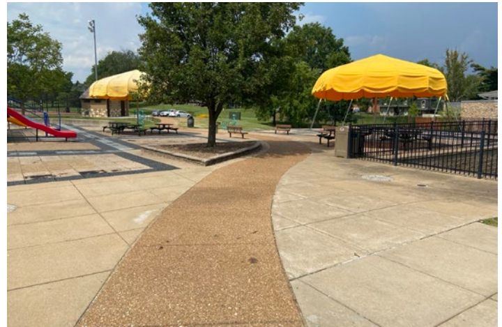
Figure 28: Concrete paths maneuver between the playground and non-operational splash pad.
