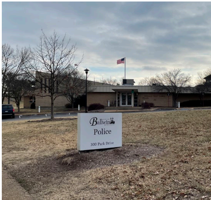
Figure 54: Police station main entrance
