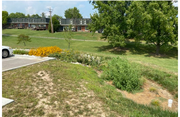
Figure 42: Bioretention cells help offset increased stormwater runoff created by impervious surfaces such as concrete or asphalt parking lots.
