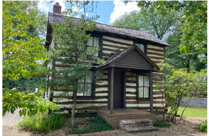
Figure 39: The Harrison-Schmidt-Dahlke Log House is a unique historic structure bringing cultural interest to the park.
