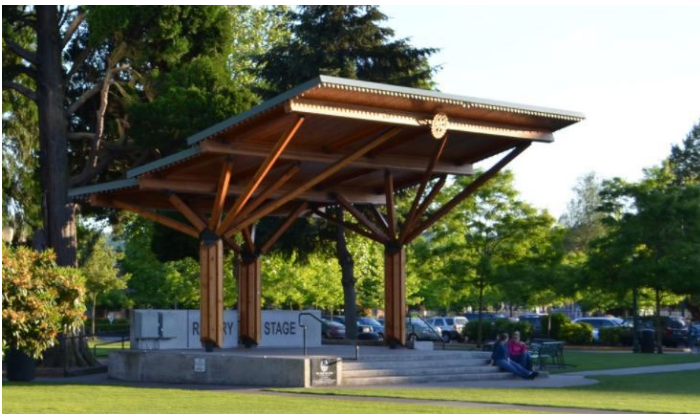
Figure 89: Example of a park shade structure.
